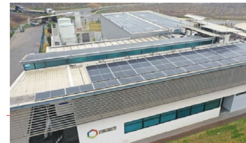
Photovoltaic system R&D Building
